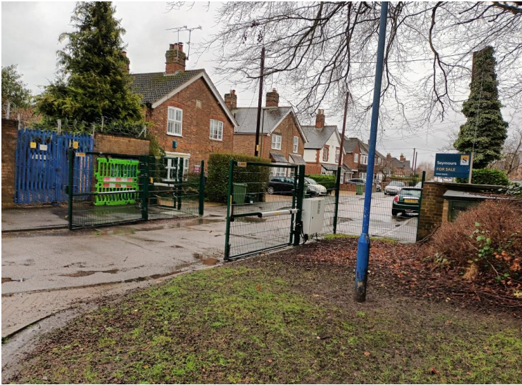
Existing southern boundary
